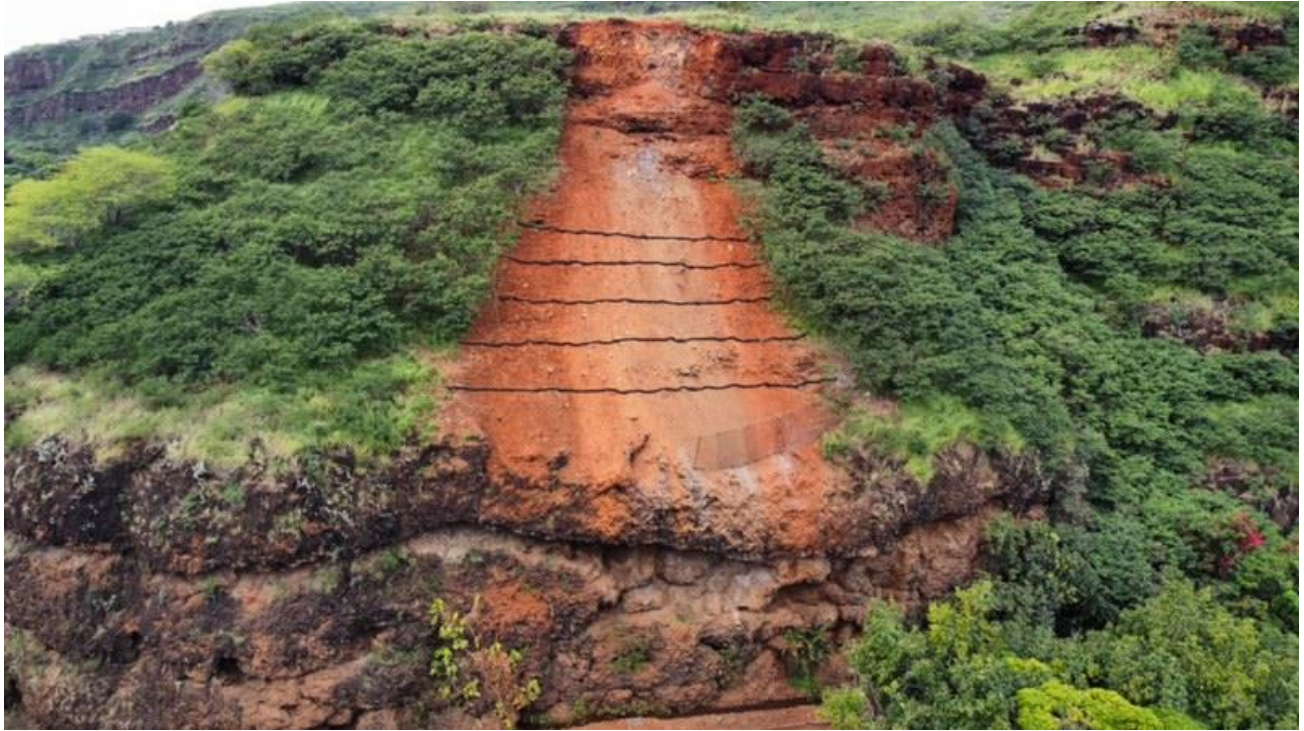
Photo caption: HiTech, the County of Kaua'i's contractor, installed erosion control measures prescribed by Geolabs – a contracted geotechnical engineering firm – on Monday, Jan. 31.
