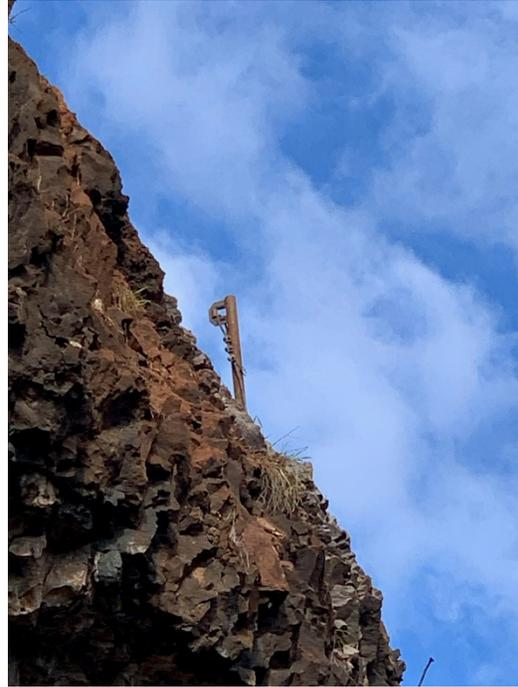
**Photo:** Contractors on Thursday began installing support posts for a chain link fence along a portion of the slope, above the Waimea Swinging Bridge. This fence will protect the bridge from rocks released during the ongoing rock scaling work. Installation of the fence is expected to continue Friday.
