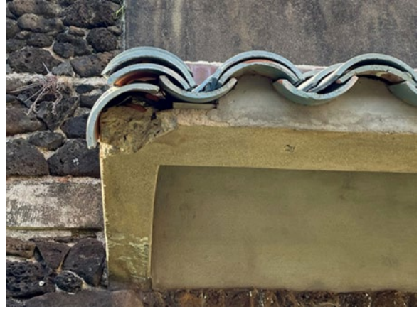
Eave Edge showing individual barrel tiles
