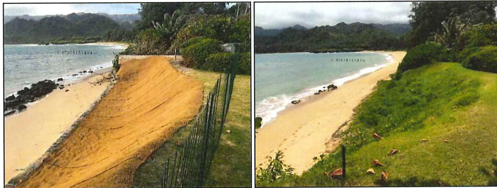
Figure 5-4 Slope stabilization with native vegetation planting on biodegradable coir providing soft shoreline protection (Lā'ie, O'ahu)
