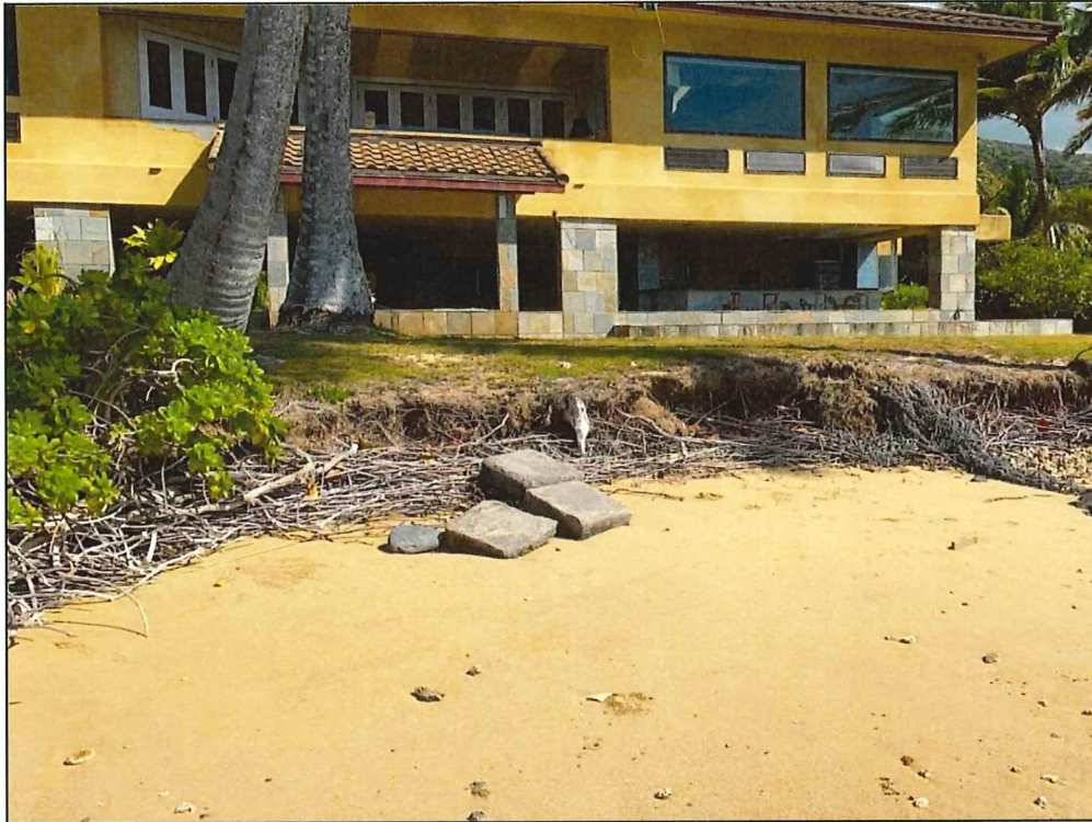
Figure 5-10 Example of vertical accommodation (freeboard) on Moloka'i
