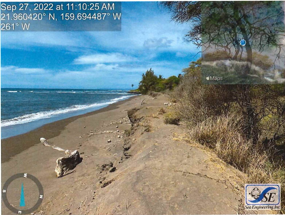
Figure 2-7: Berm fronting the study area with an erosion scarp along the seaward edge
