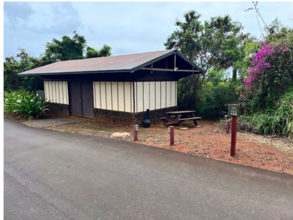
10. Existing Building near Proposed ADA and EV Parking
