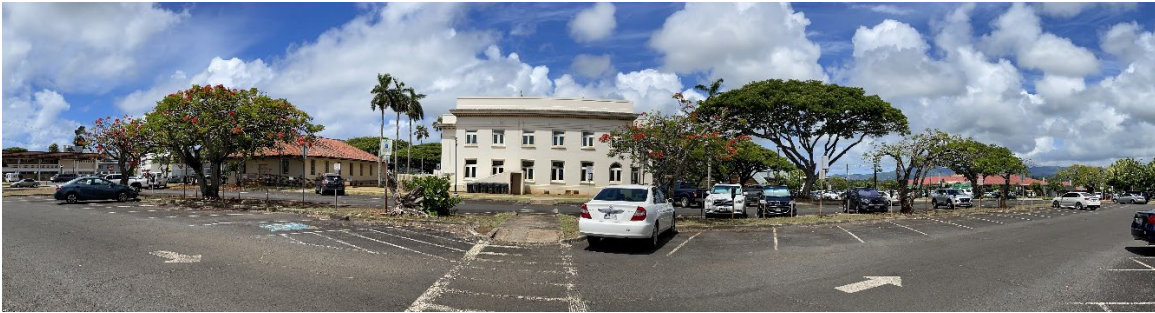
Existing parking lot at Mobility Hub site
