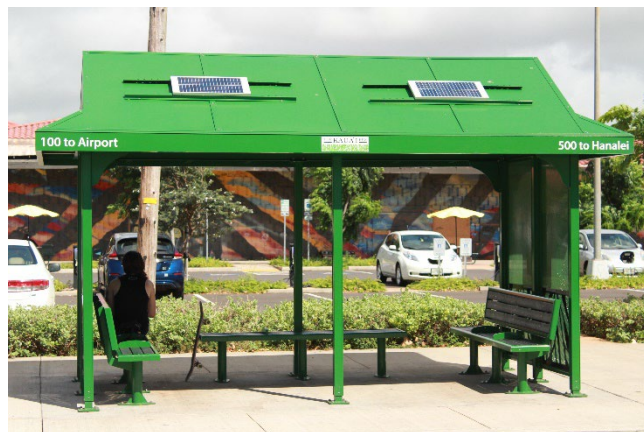
Kaua'i bus shelter with solar panels.
