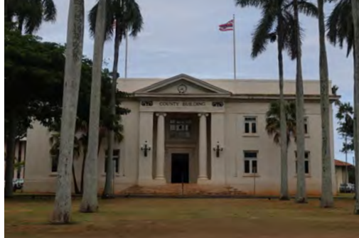
View of Historic County Building from Rice St.
