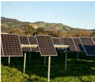
Example of solar panel grid supply
