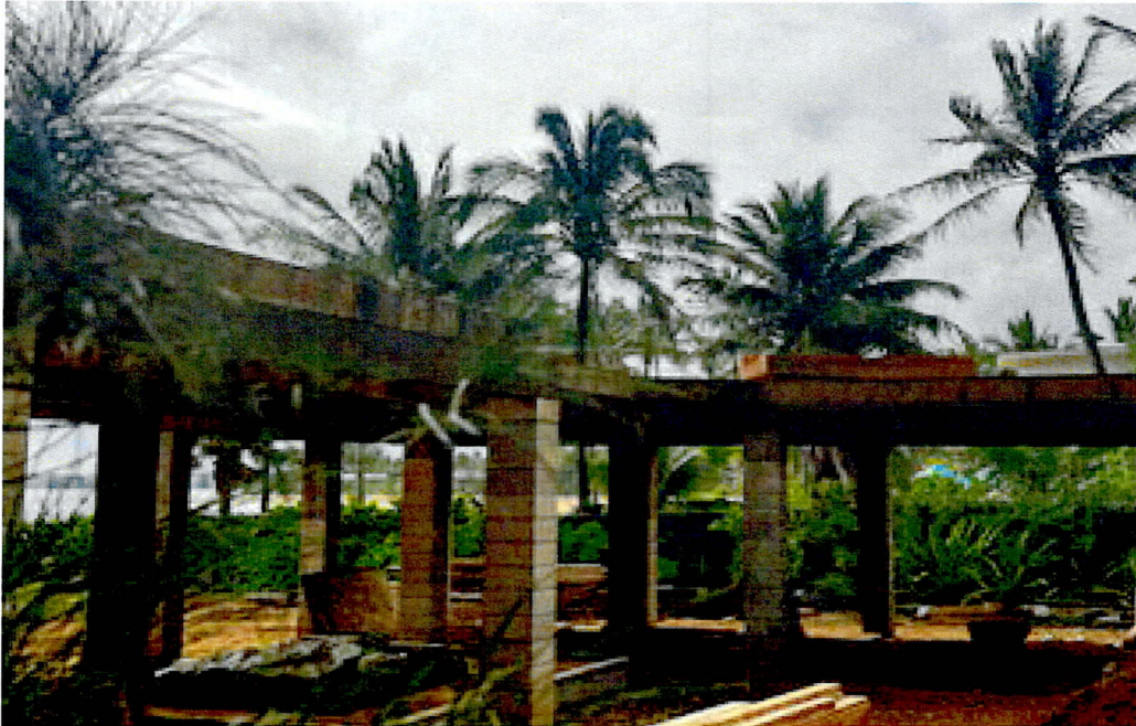
Photo 3 dated July 13, 2024 shows the house gone, minus the new footing columns.
